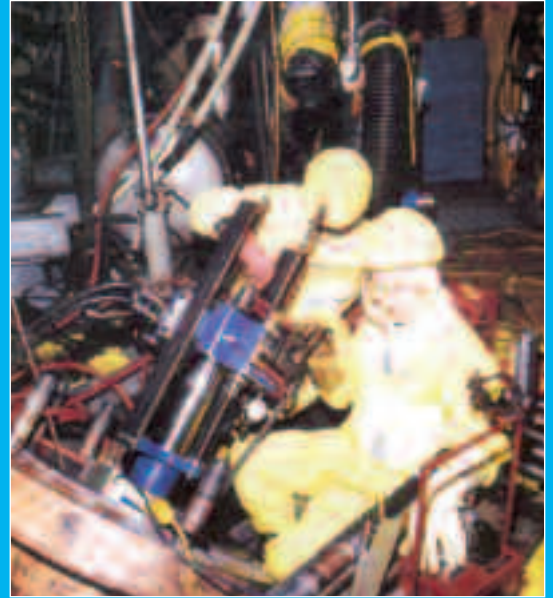
MSIV repair in containment at Nuclear Plant
