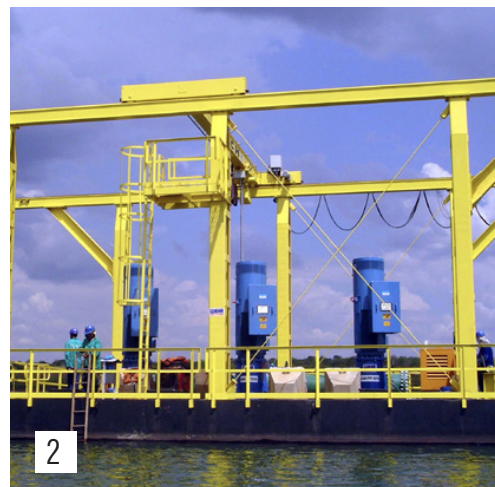
1: 2000 HP raffinate pumps 2: Reclaim water pumps 3: Tailing water pumps
