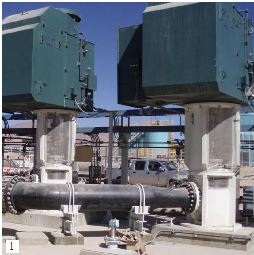
1: 2000 HP raffinate pumps 2: Reclaim water pumps 3: Tailing water pumps
