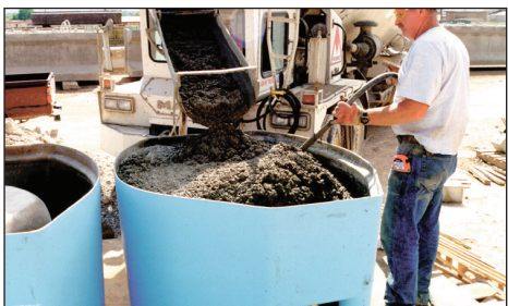
Step 4: Fill shell with concrete mix.
