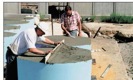
Step 6: Settle and level base of fiberglass shell, allow concrete to cure.
