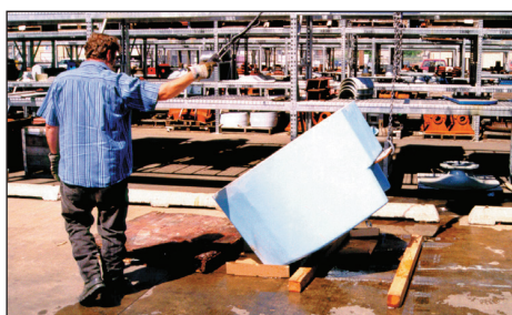
Step 8: Place protective surface in appropriate location before turning concrete filled basin right-side up.
